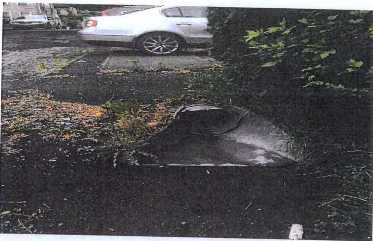
Outfall No. 3 – 15 inch corrugated metal pipe discharge to canal – end of Jefferson Street
